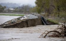
CALIFORNIA DEPARTMENT OF WATER RESOURCES After a March 11 levee failure drowned Floodwaters from the Pajaro River flow through a levee break near the township of Pajaro in Monterey County on March 12.
